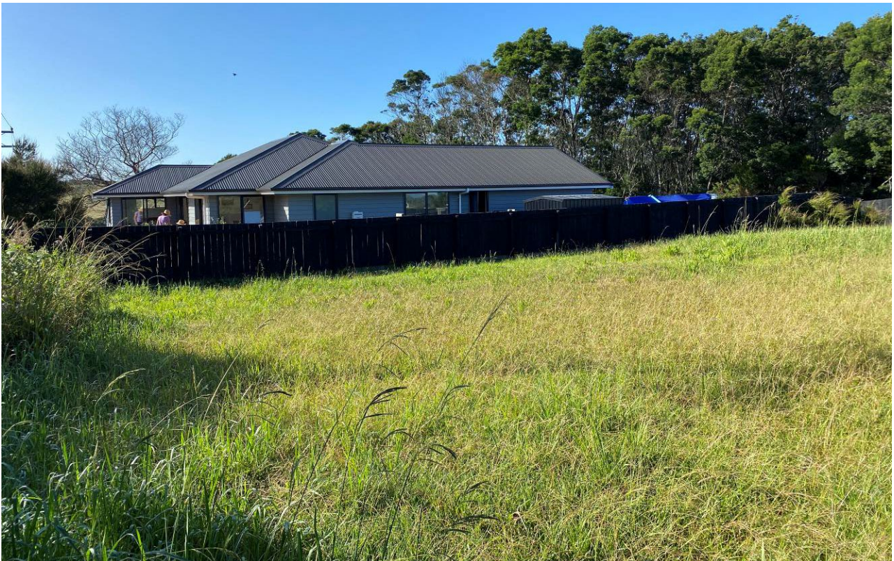
Photograph 2 showing an existing 1.8m high wood fence providing a reasonable level of privacy to neighbours to the east. The owners of the eastern property have planted shrub species and cabbage trees to provide privacy for them while they use their deck area.
