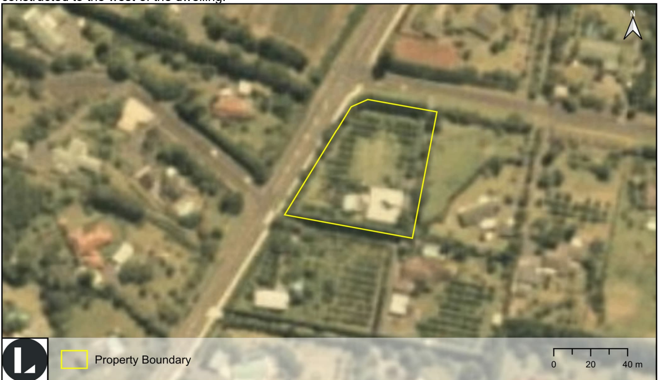
Figure 15. Aerial imagery 2000. Sourced from LINZ (annotated image). Approximate site boundary shown in yellow.
