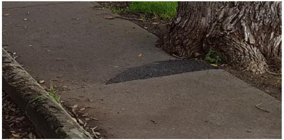
Fig 1 – The buttress roots of this tree have lifted the concrete footpath (creating a trip hazard)
