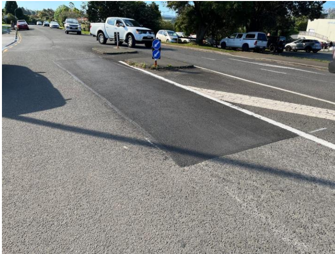
Butler Road Mill and Fill
