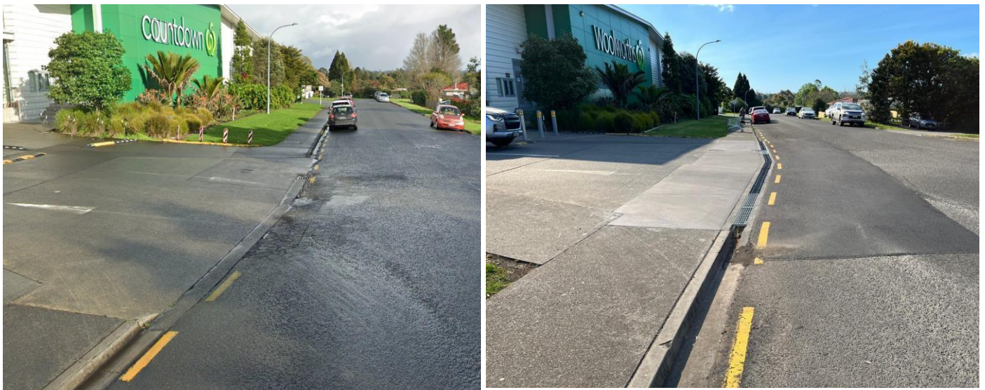
Butler Street before / after
