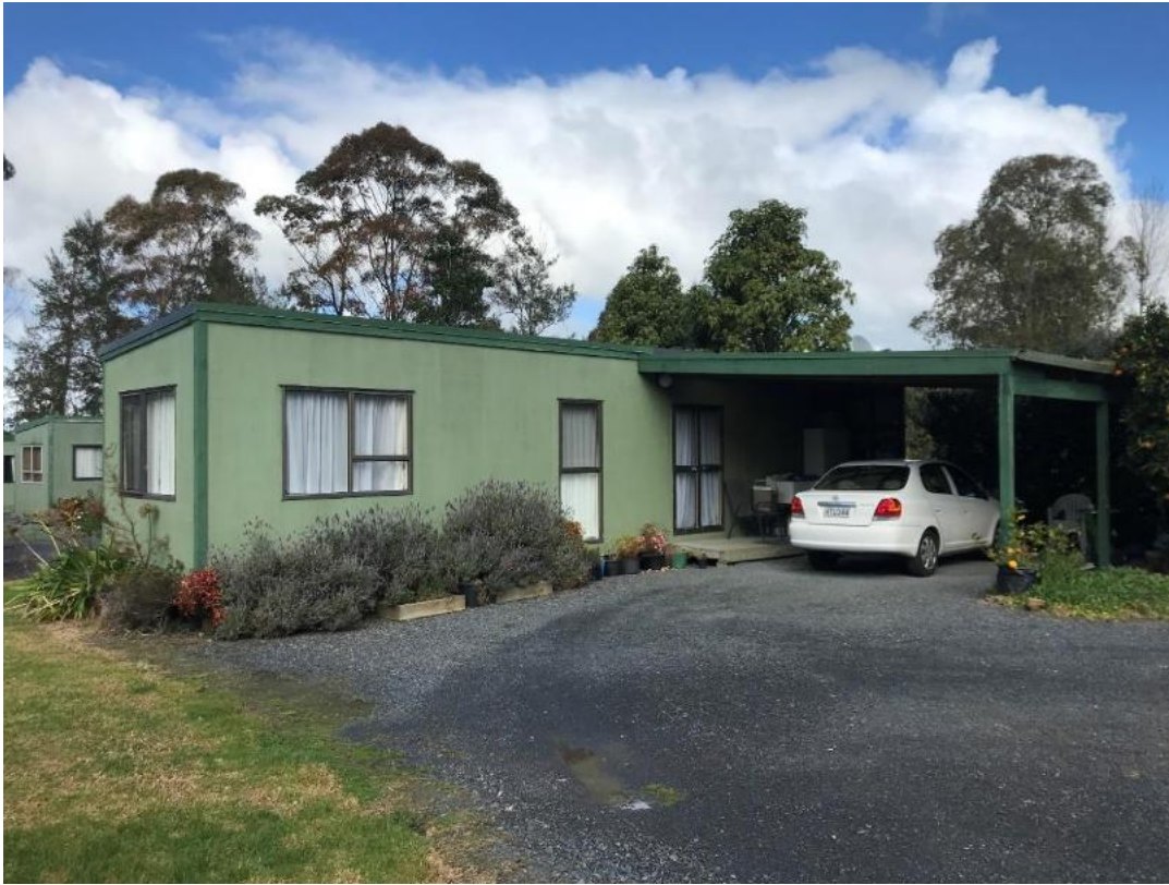
Figure 14 - Existing residential units on site
