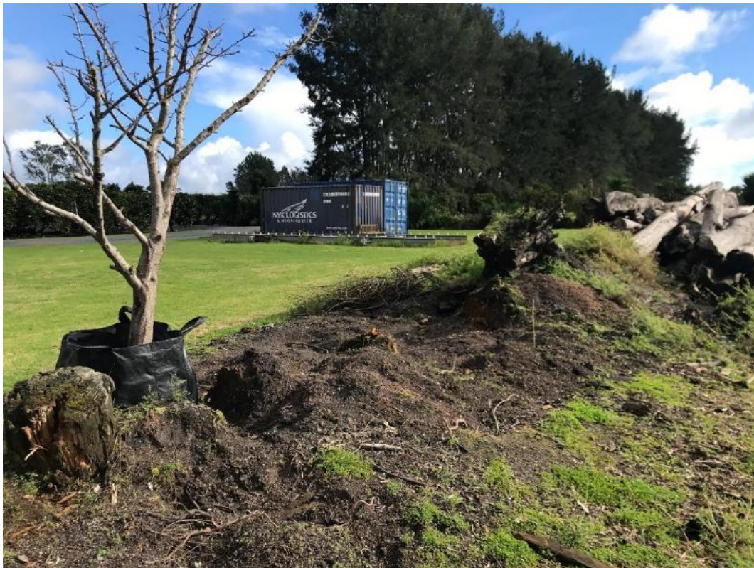
Figure 13 - Central strip of felled materials and natural burn pile
