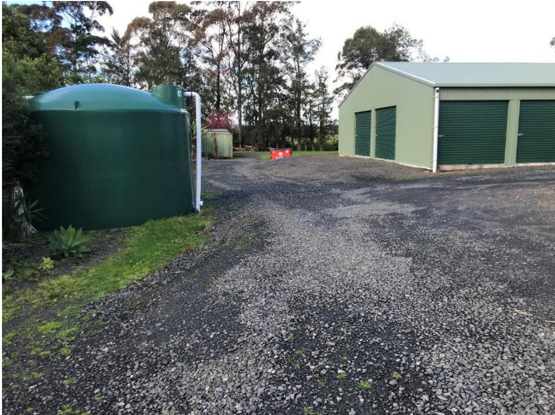
Figure 18 - One of the 30,000 L water tanks
