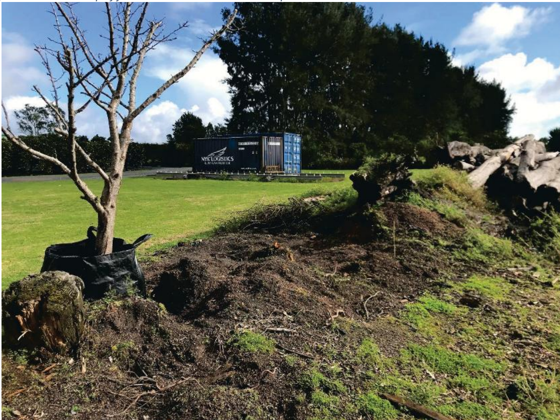
Figure 36 - Central strip of felled materials and natural burn pile
