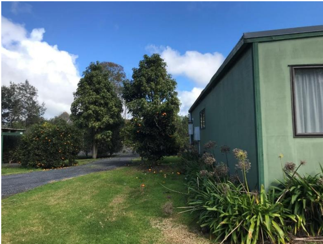
Figure 15 - Existing residential units on site
