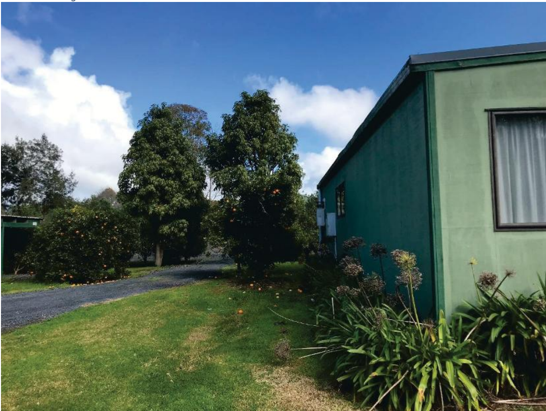
Figure 44 - Existing residential units on site
