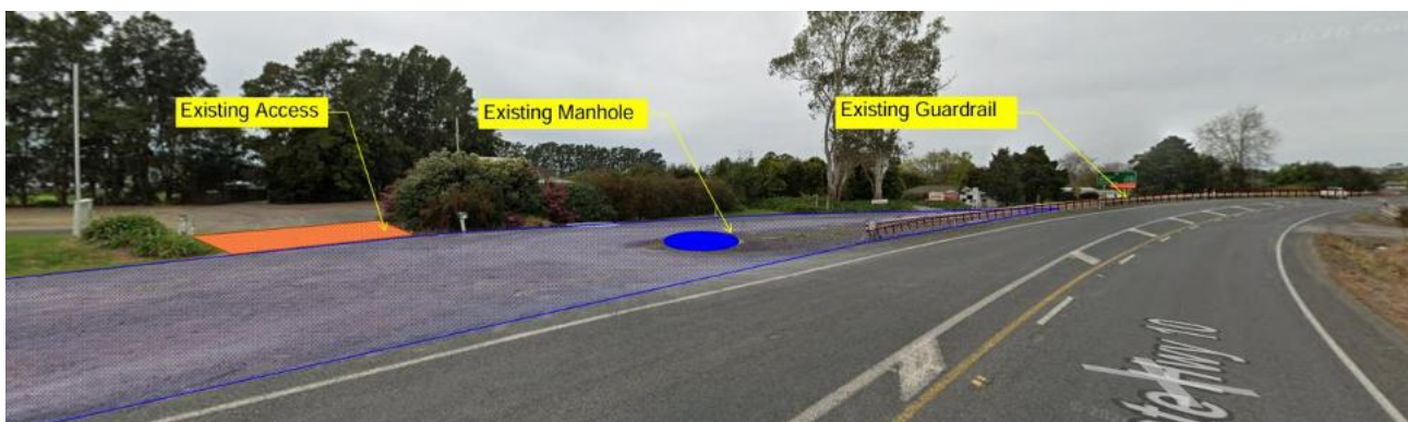
Figure 13: Location of Access in Relation to the Manhole and Guardrail
