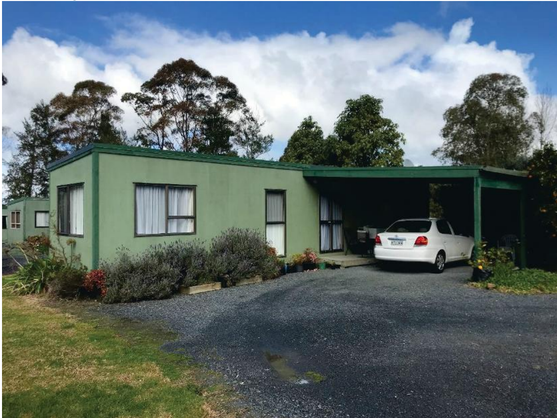
Figure 43 - Existing residential units on site
