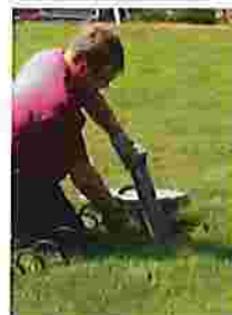
Lifting and hosing down effluent outlet filter
