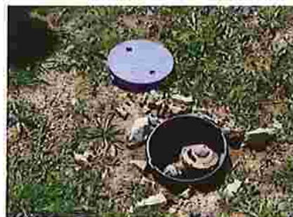
Automatic sequencing valve
