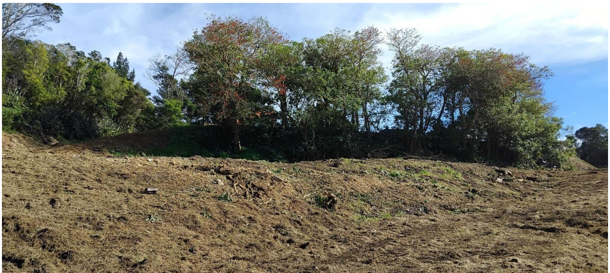
Figure 10 - View from the mid-point of the landfill facing the upper portion of the landfill cell.
