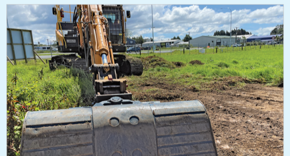
Construction begins on the new multisport complex at Waipapa.
