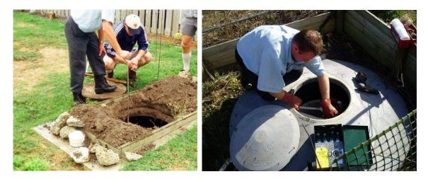
Checking scum and sludge levels in a septic tank
