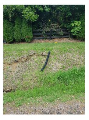
Existing overflow outlet from water tanks
