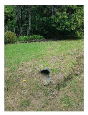
450mm culvert from open drain into Pa Rd swale
