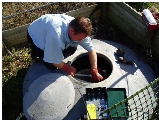
Servicing an advanced wastewater treatment unit
