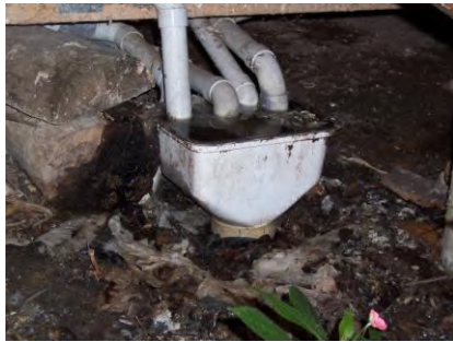
Backup to gully trap from clogged tank
