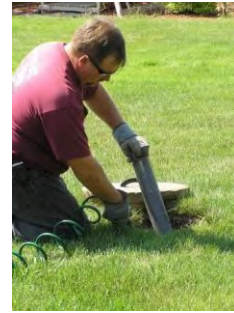
Lifting and hosing down effluent outlet filter
