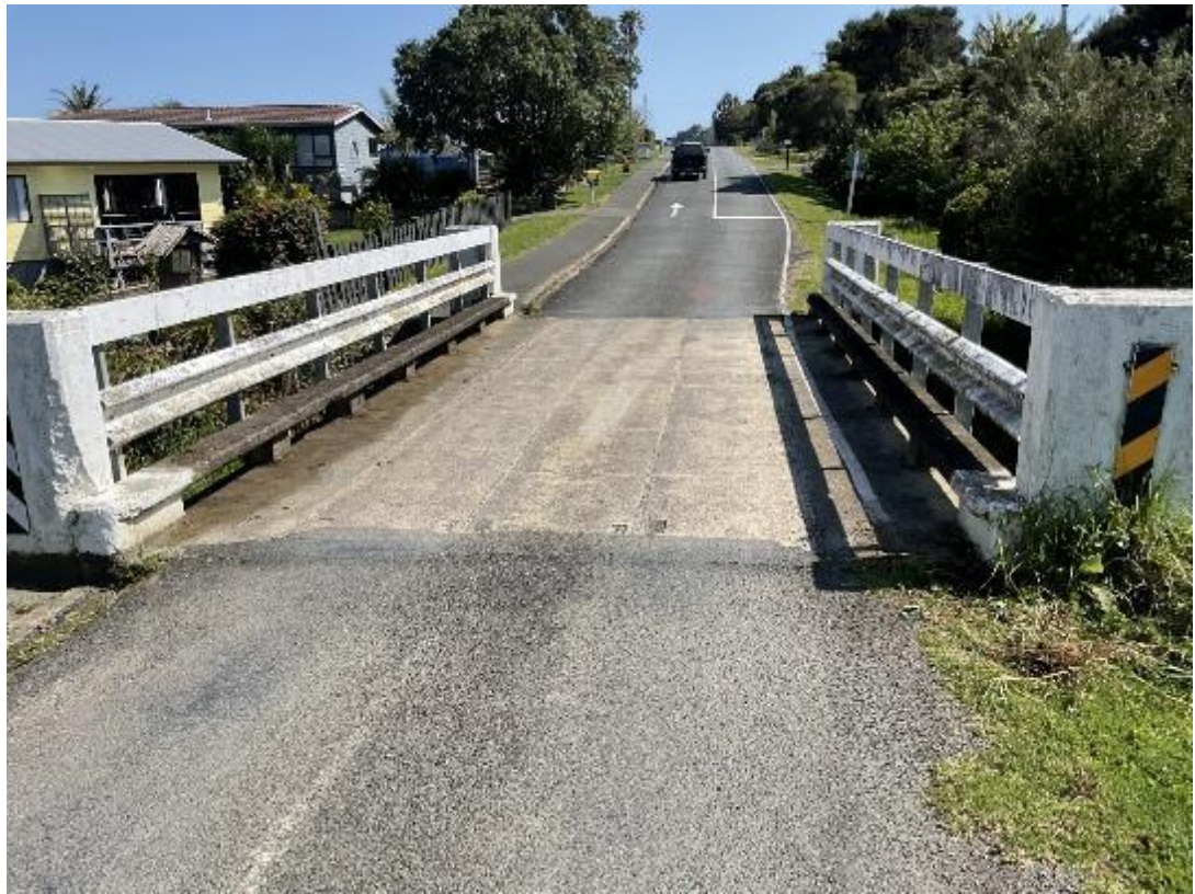
Hihi Beach Rd – Bridge Deck Clearing
