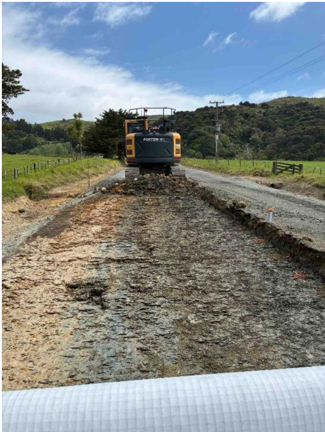
Hihi Rd Rehab – Pavement Undercuts in Progress
