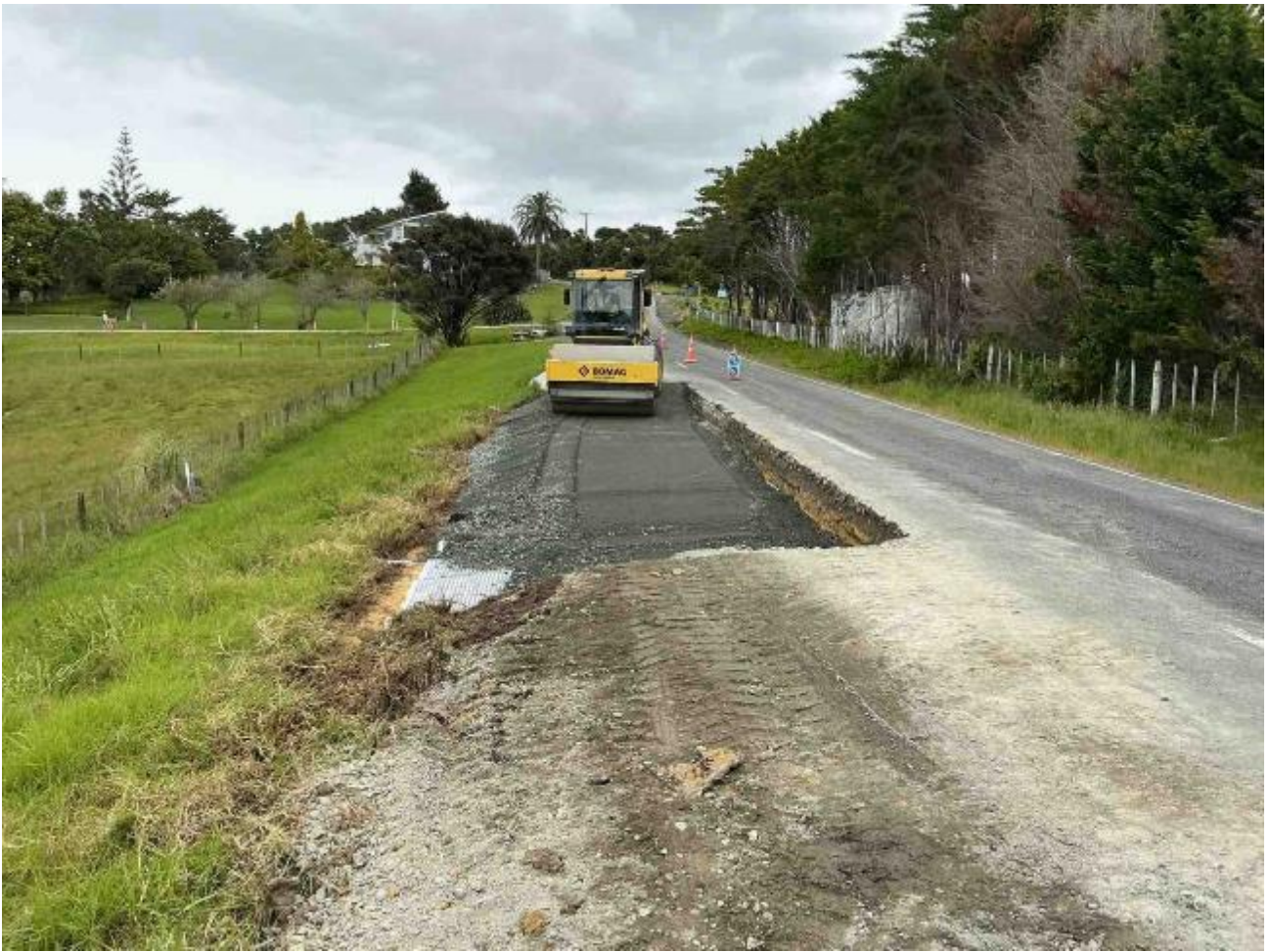
Taipa Heights Rd – Digout Repair in Progress
