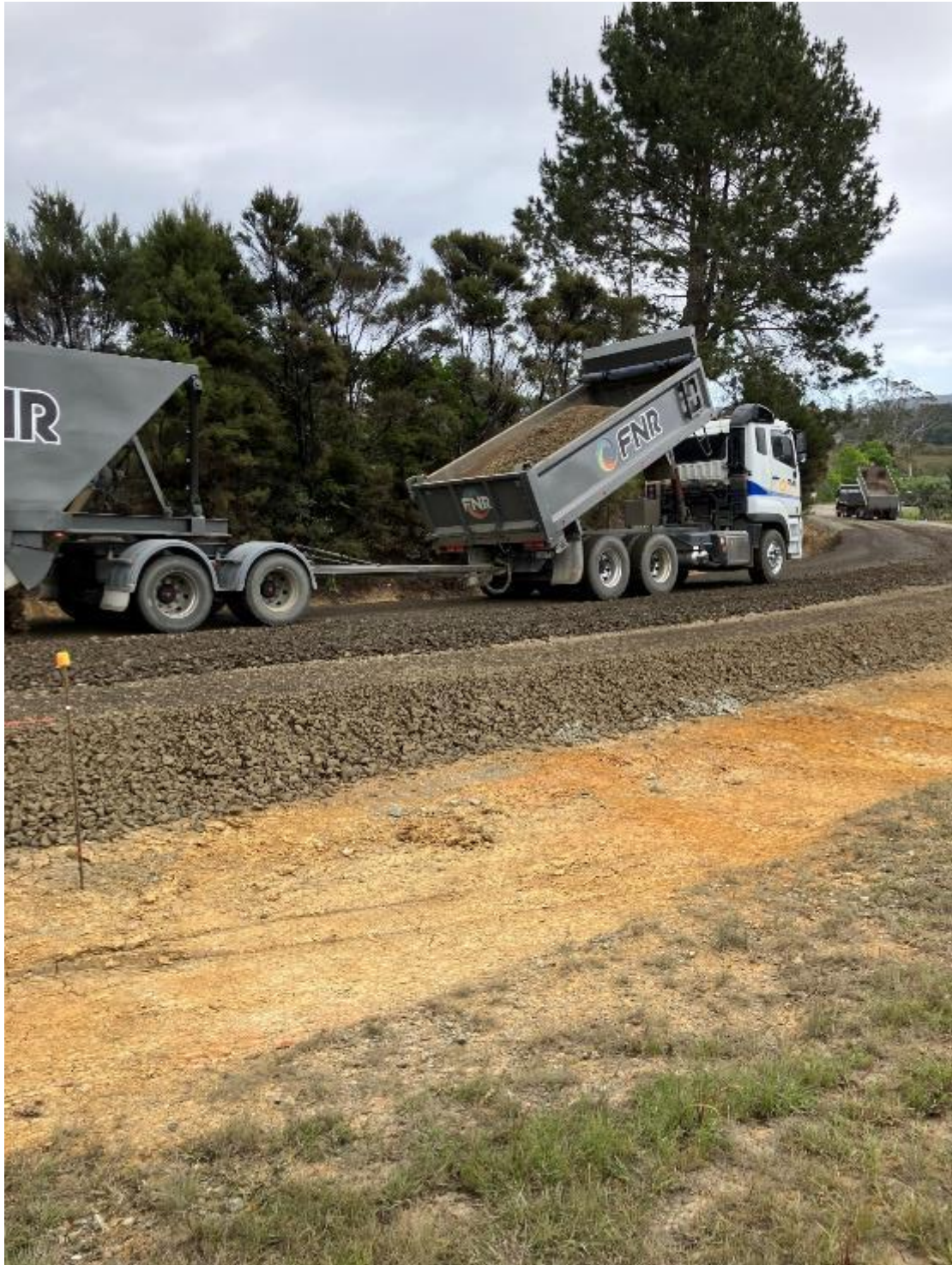
Hihi Rd Rehab – Pavement Overlay in Progress
