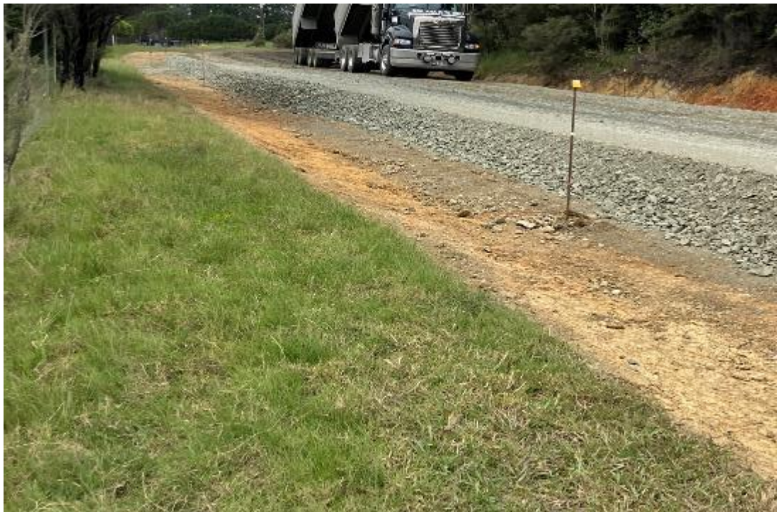
FNR trucks hauling metal for the Pavement Overlay – Hihi Rd Pavement Rehabilitation
