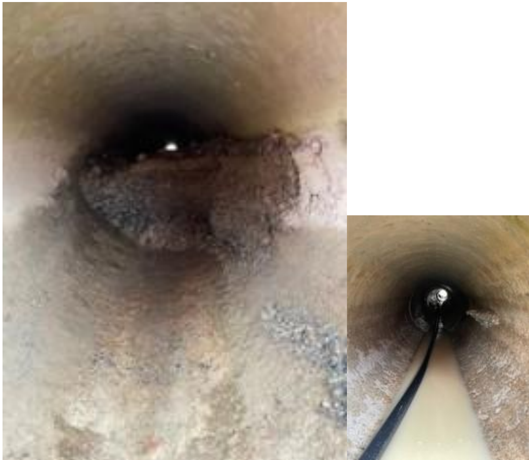
Pupuke Mangapa Rd – Culvert Flushing Before and After
