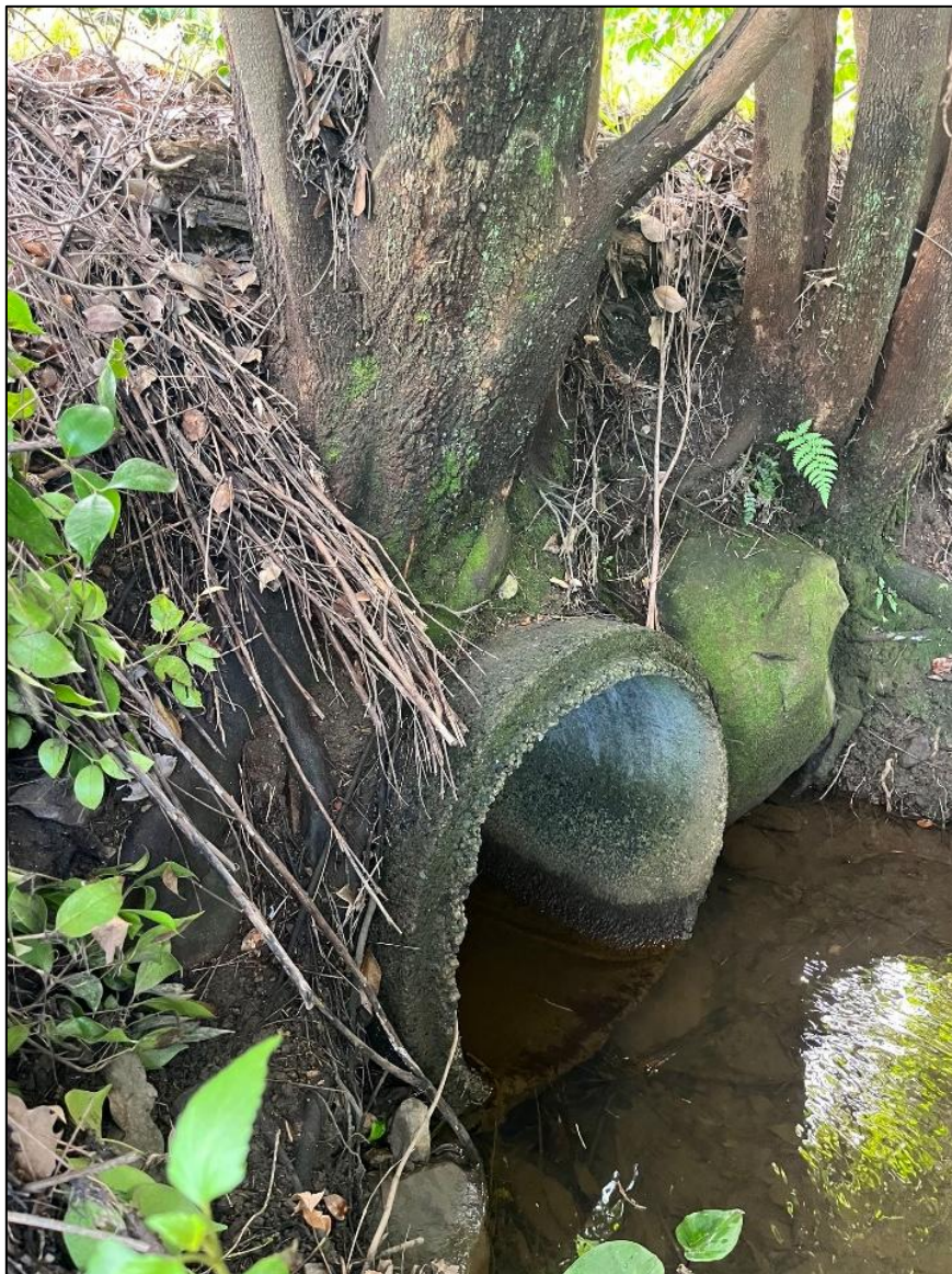
Figure 6: 12.06.2025 Site Photo – View of existing 600Ø culvert in stream under existing accessway.
