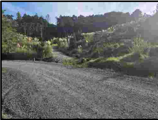
Figure 4: Image of existing access to Lots 1, 2 & 3, which will be upgraded to Council standards.
