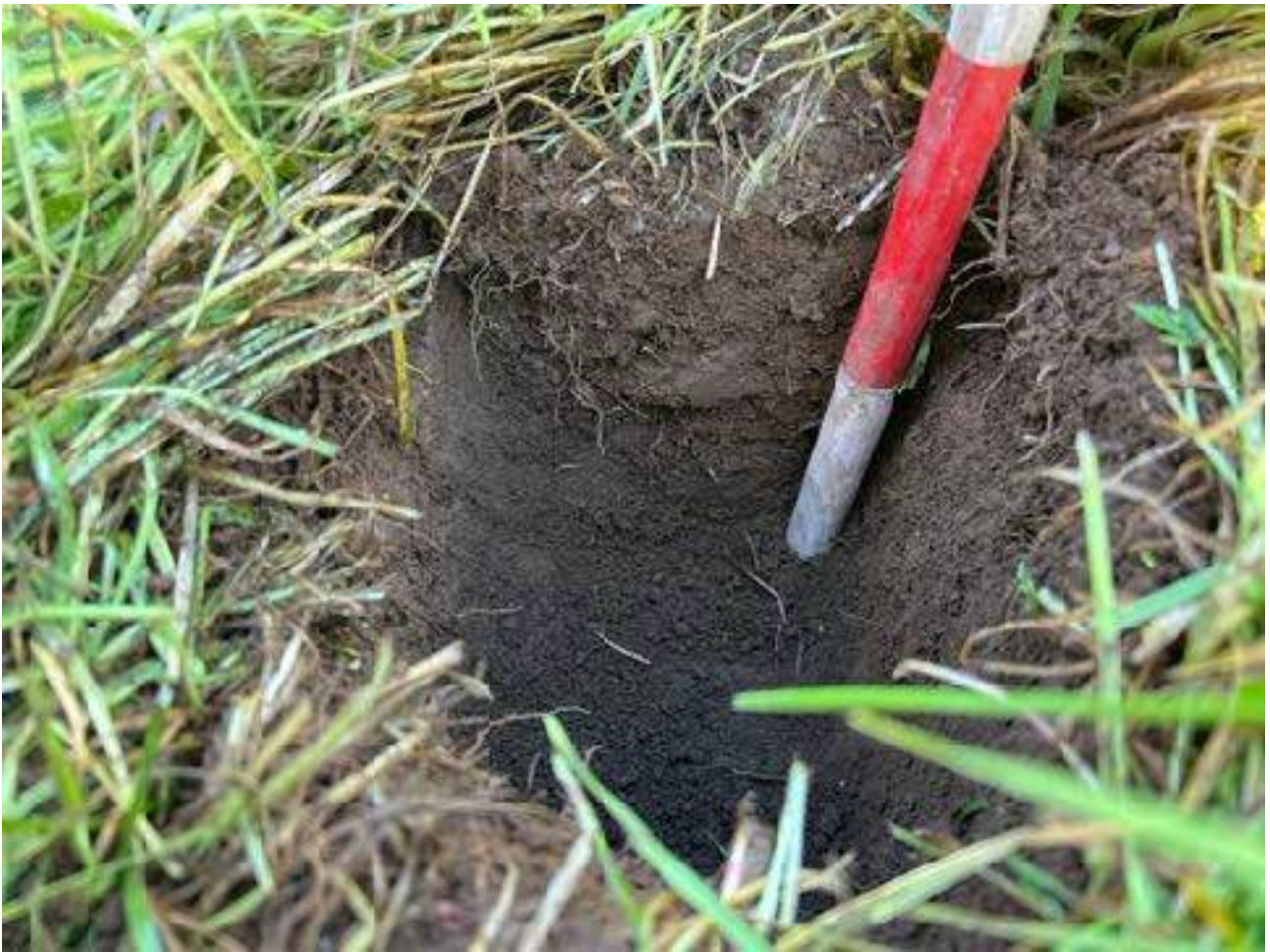
Figure 22. Detail of Test Pit 2 (within proposed building envelope)
