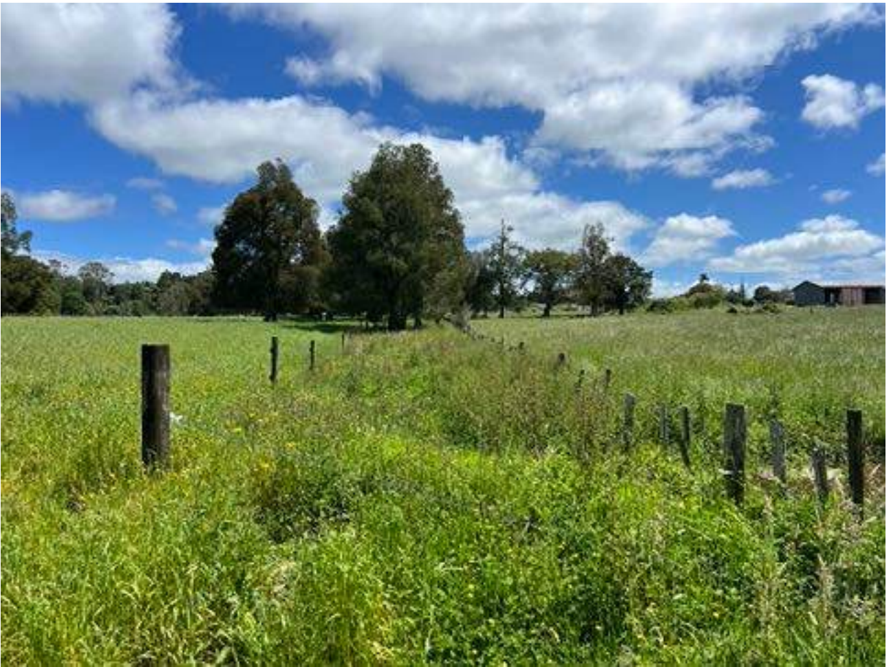
Figure 37. View north over cut drain within Proposed Lot 8
