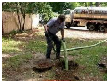
Septic tank pumpout
