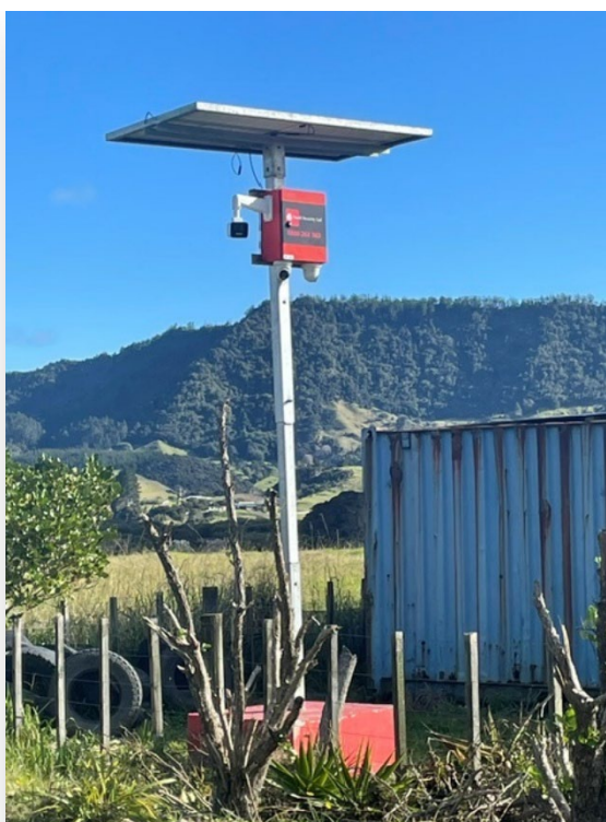
Figure 13 - Camera installed at Herekino Transfer Station
