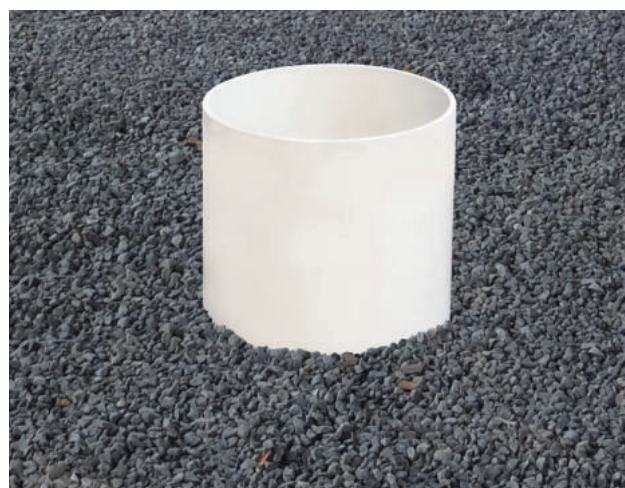
Fig. 17 Install port into RainSmart System
