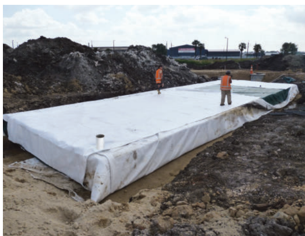
Fig. 16 Installed maintenance port
