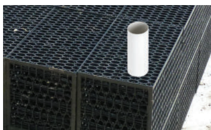
Fig. 11 Installed inspection port.
