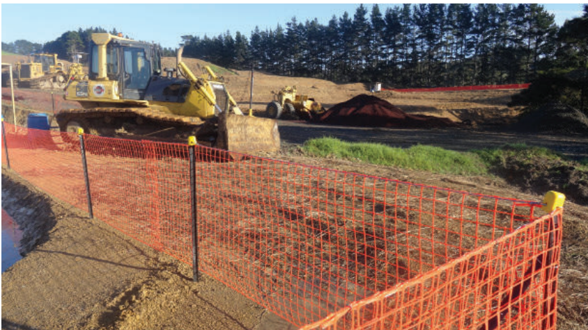
Fig. 25 Secure RainSmart system installation using barriers.
