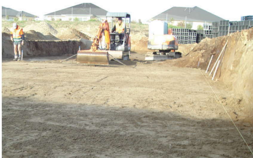
Fig. 5 Base must be smooth to ensure modules fit together without gaps.
