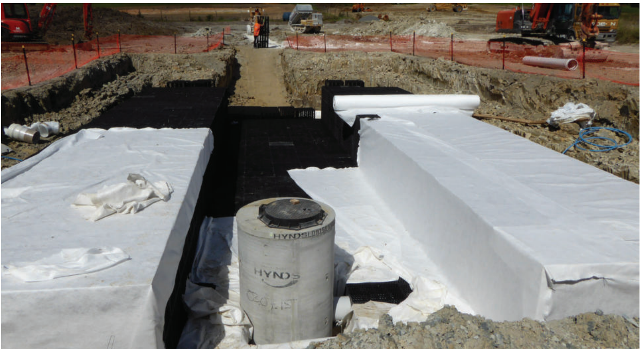
Fig. 18 Encapsulate RainSmart system with geotextile
