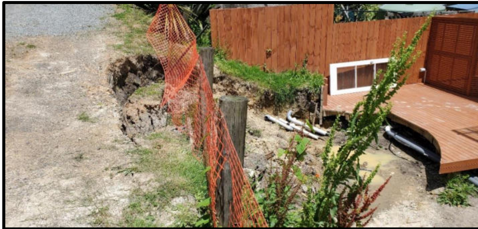
Figure 29: Slip which has occurred during a rain event where it has affected the neighbouring allotment (Allotment 2A).
