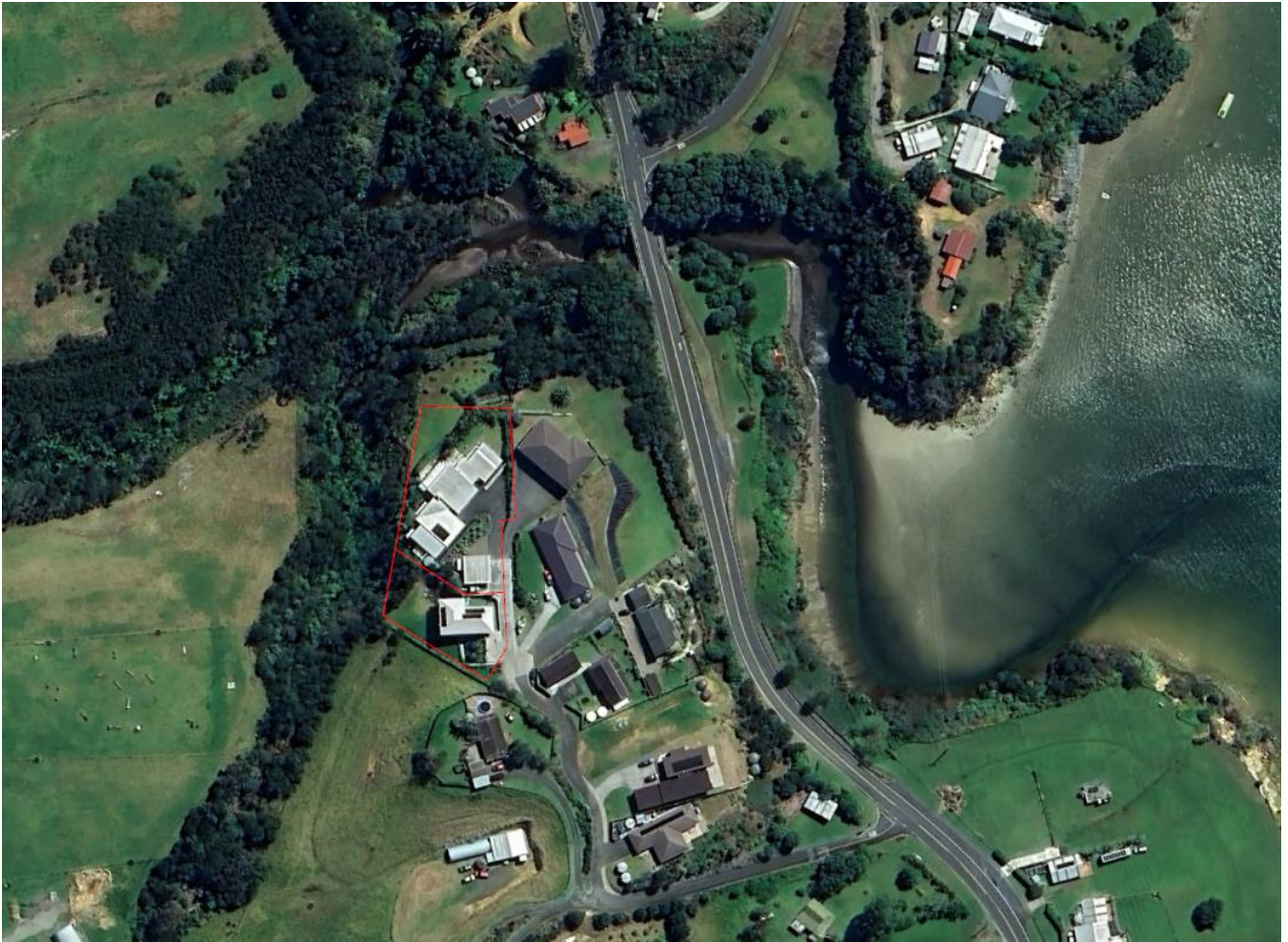
Figure 2 – Aerial Photo Overview
