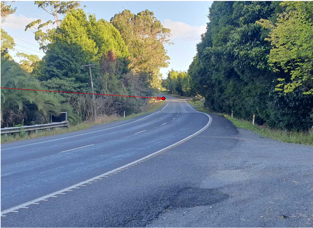
PHOTO FROM DRIVEWAY, NORTH OF DRIVEWAY CROSSING
