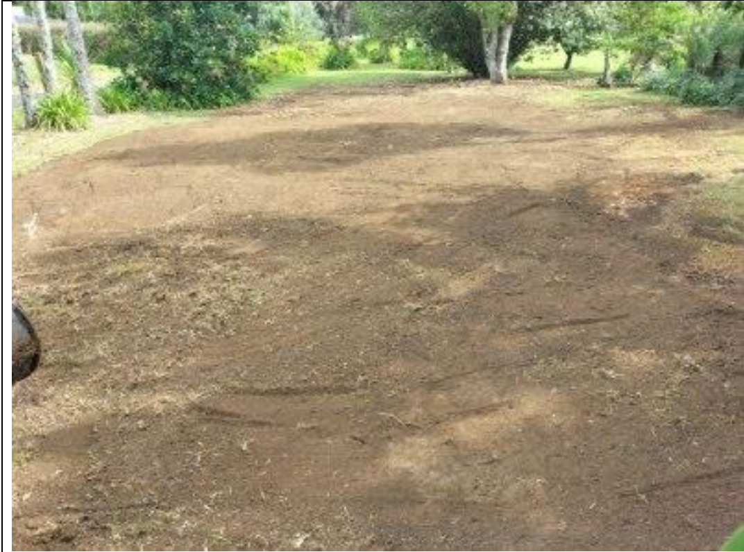
9. Topsoil backfill of remedial cell.
