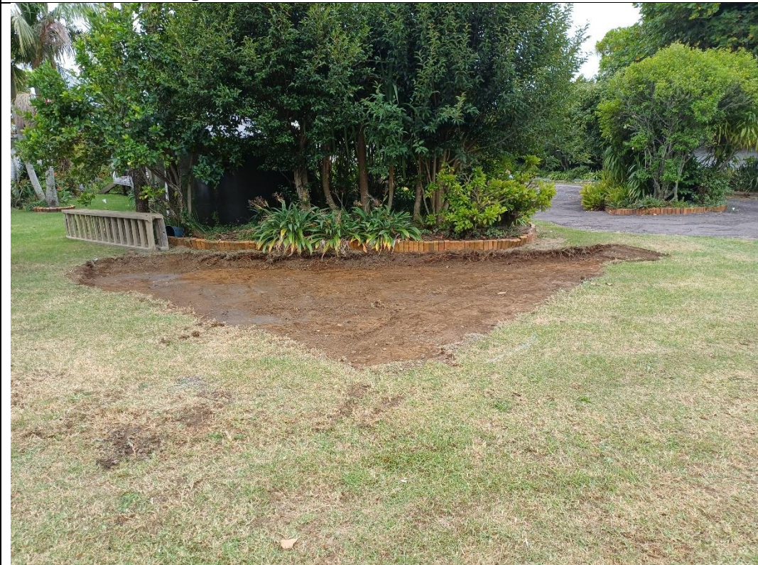
2. ES34 remedial excavation
