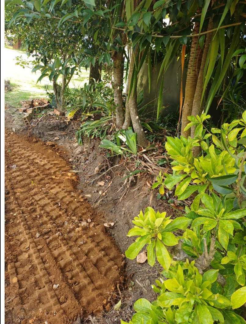
6. Additional excavation to ES34
