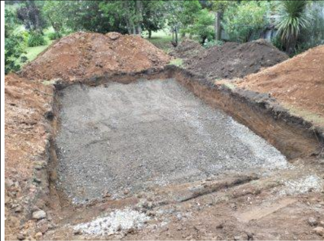
7. GAP65 aggregate no dig layer placed in remedial cell
