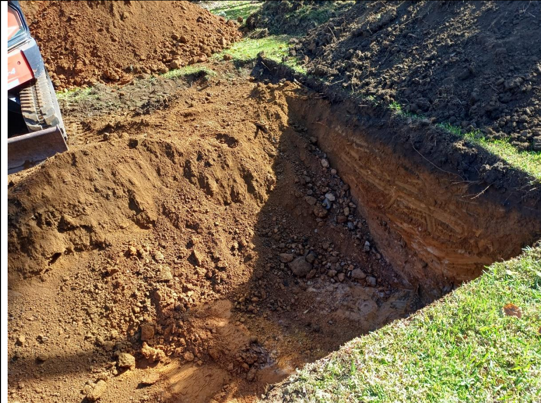
1. Remedial cell being excavated.
