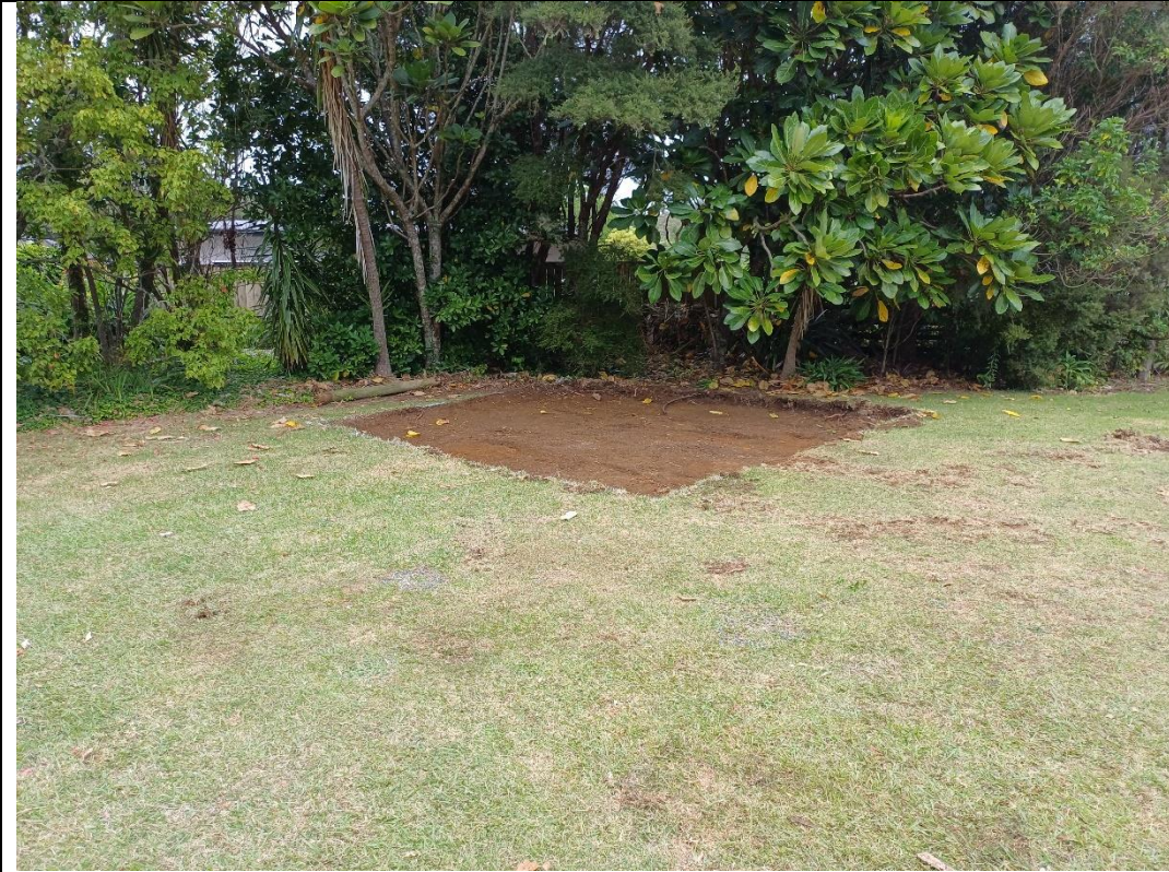
5. Remedial excavation ES3
