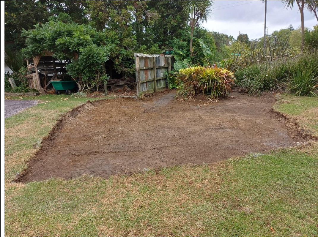
3. Remedial excavation ES1
