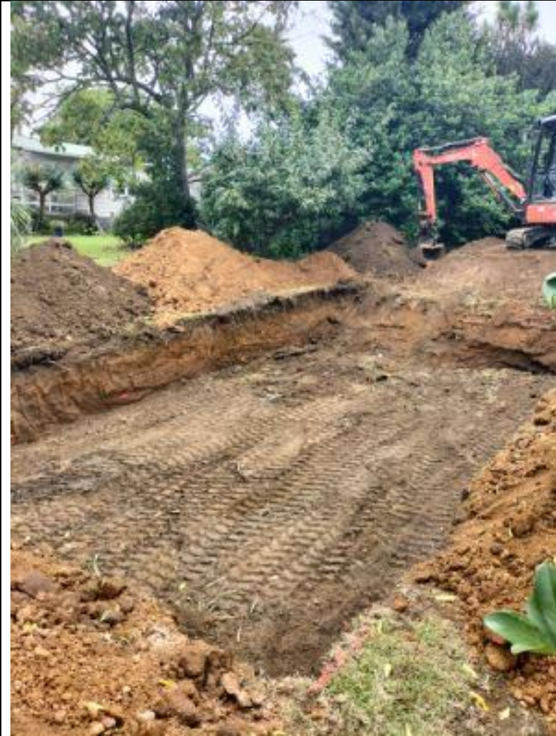
8. Subsoil backfill in remedial cell.
