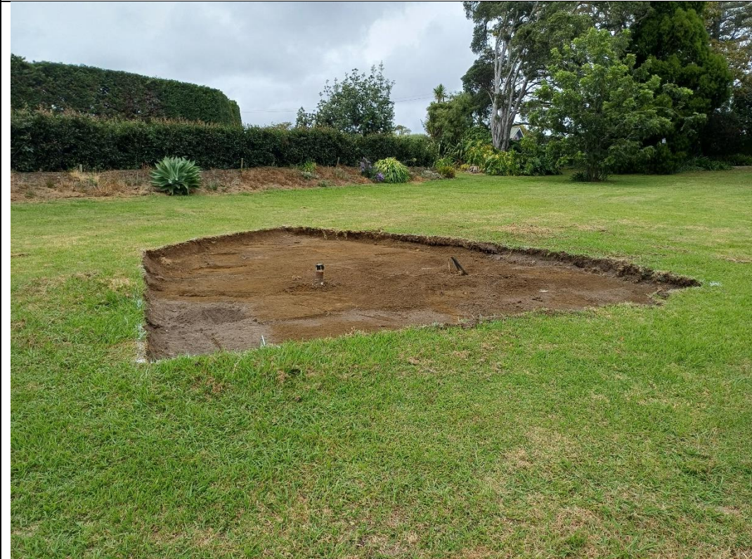
4. Remedial excavation ES11
