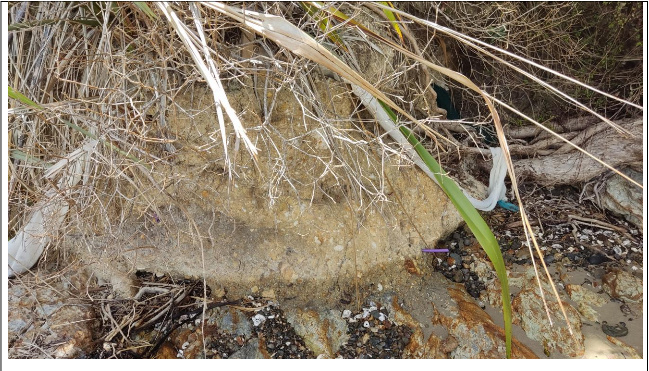
Figure 7 – Slip material at base of bank with debris from the former wastewater field.
