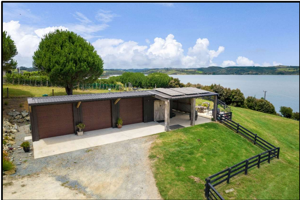
Figure 10: Image of the subject shed showing colour scheme as well as the siting of the shed into the existing landscape.
