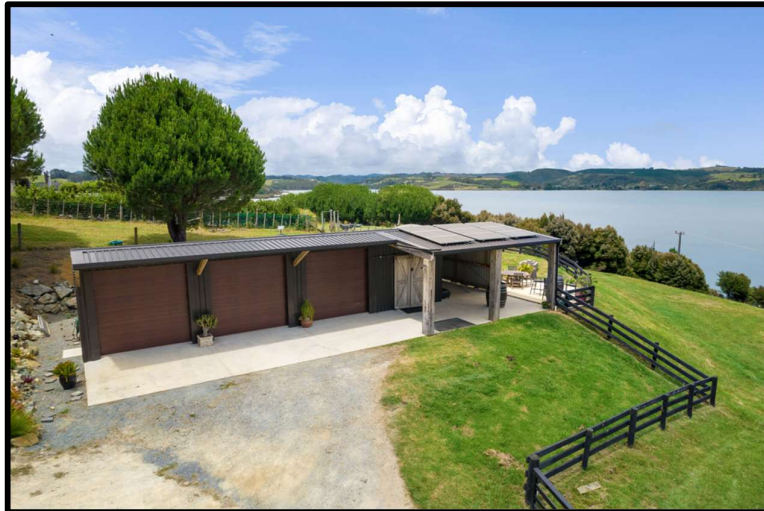
Figure 2: View of Shed from within the site
