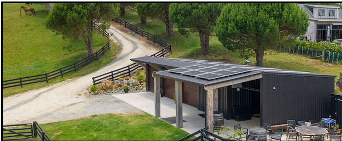
Figure 3 - Shed with neighbouring dwelling in background
