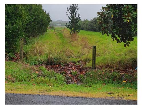
75. Indeed the lack of maintenance of the drain opposite 104 Waitotara Drive results in the storm water ponding the road swales and then overtopping across the carriageway just in a typical couple days of rain!
