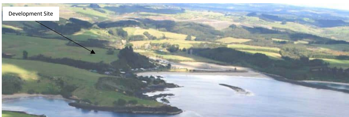
Figure 12. Oblique Aerial of Site Courtesy Northland Regional Landscape Assessment Worksheet dated February 2014.
