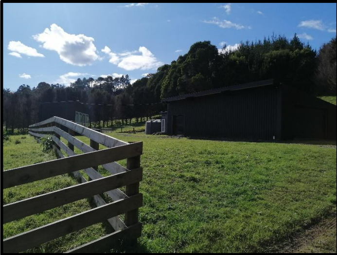
Figure 9: Existing shed, utility units and sleepout on Lot 1.
