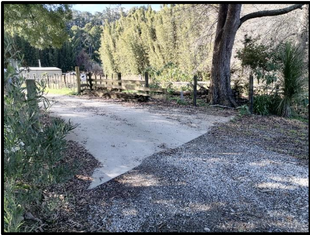
Figure 6: Existing access to Proposed Lot 2.
