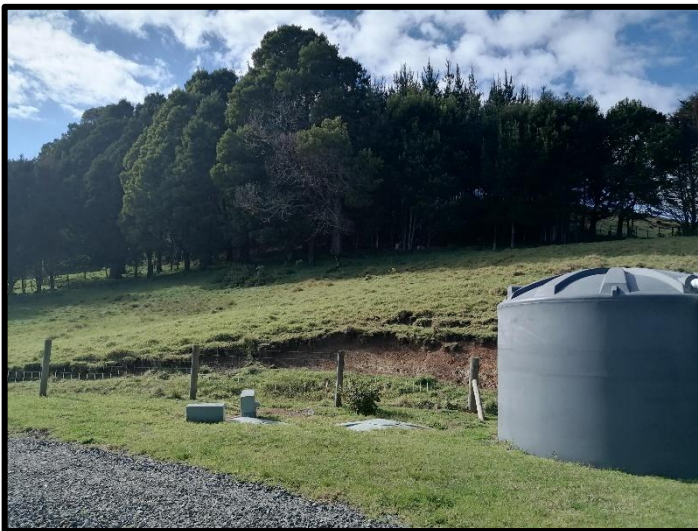
Figure 12: Existing water tank and septic system on Lot 1, located to north of buildings.
