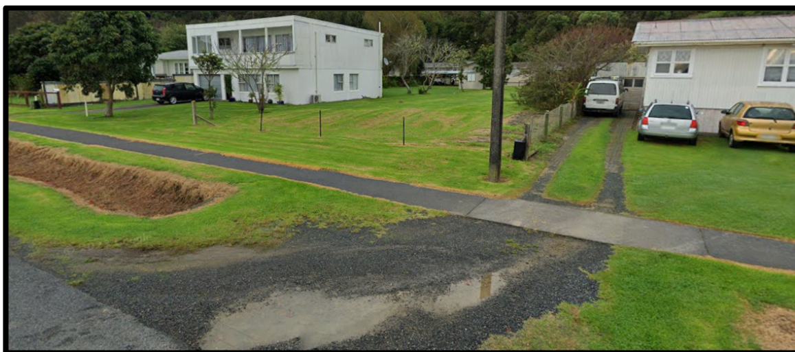
Figure 3: Image showing existing vehicle crossing to subject site (Google Streetview)
