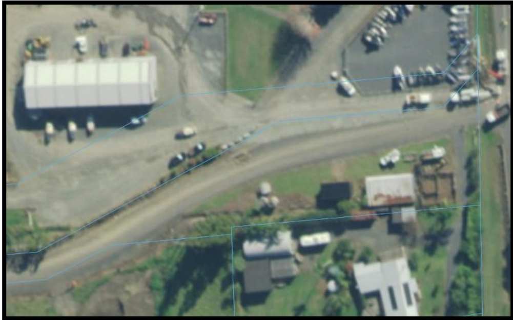
Figure 4 - Aerial view of driveway locations in relation to property boundaries.
