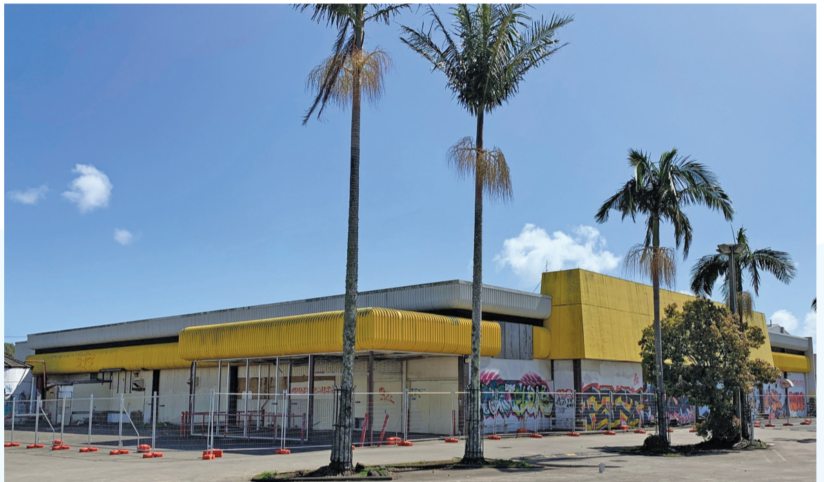
Works around the carpark will be carried out in conjunction with the Te Hiku Working Group as part of the Te Hiku Revitalisation Project.
