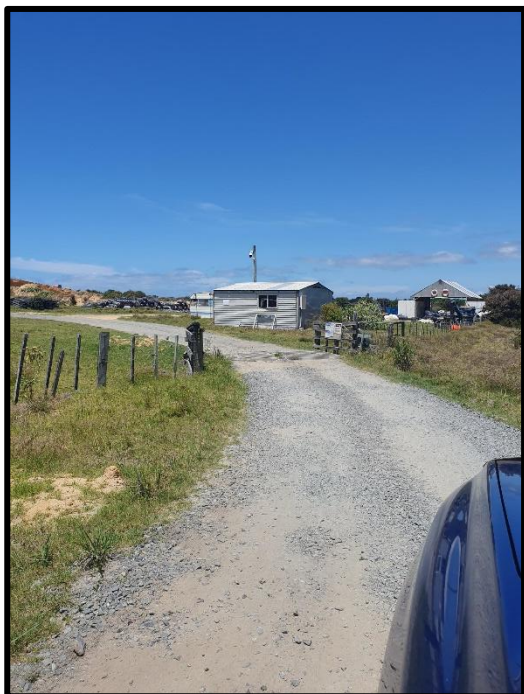
Figure 5: Internal drive to the existing dwellings on Lot 2.
