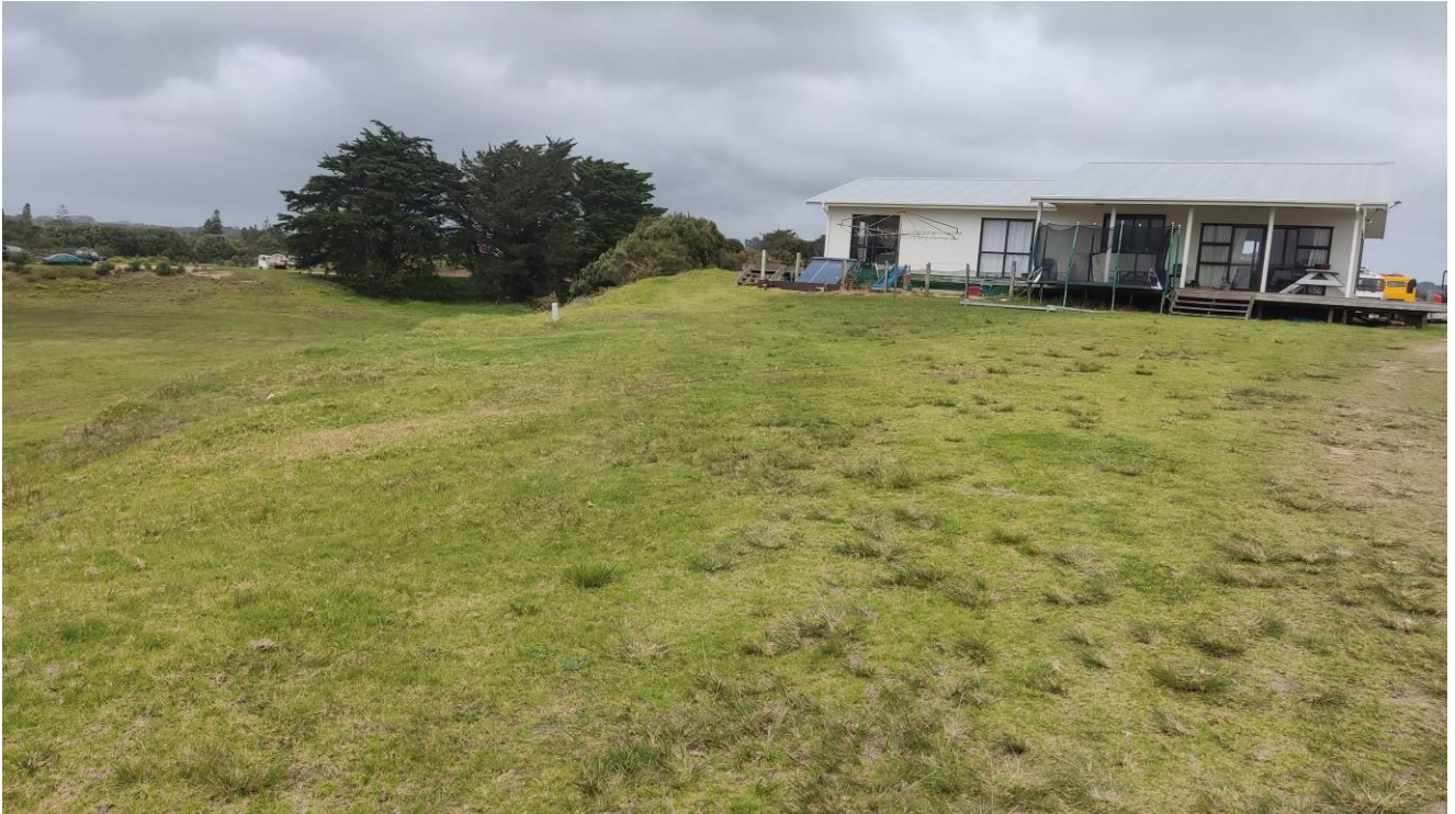
Figure 10 Wastewater treatment system and disposal area for southwestern dwelling on proposed lot 2
