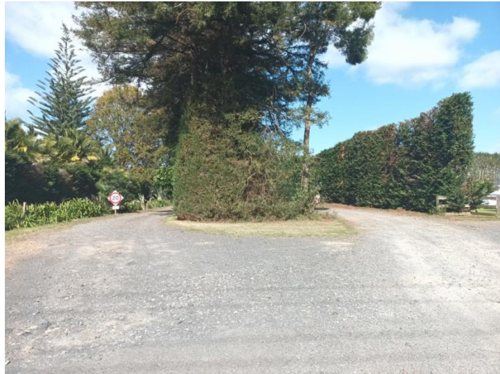
Looking south from crossing off KC Inlet Road. Left hand fork (eastern), with speed restriction signs and speed humps; and right hand fork (western) previously used by NTW traffic
