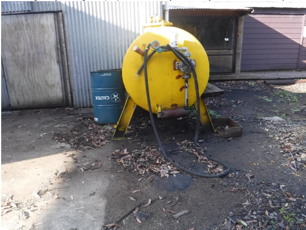
Figure 8 – Above ground fuel storage tank (AST) situated to the adjacent north of the wood mill within the yard.
