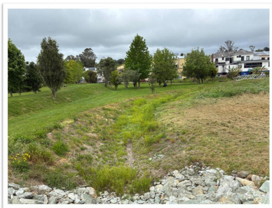
Photo 24: The existing stormwater swale along the east flank of the proposed site.
