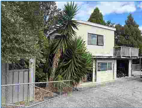
Photograph 2: Existing garage / storage building. Car deck to be formed to the east of the building, selected removal of mainly exotic vegetation required. Upper-level addition upon existing deck.
