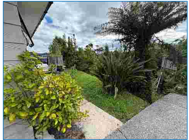
Photograph 3: Location of existing lawn to be filled to form a retained and level lawn area.
