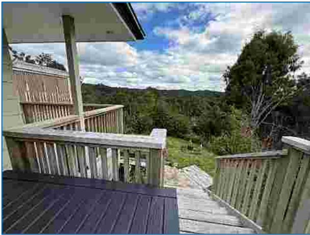
Photograph 1: Illustrates the western end of the existing dwelling, the small playroom to be removed, and the existing grass area upon which the house addition and part of the pool / deck addition will be located.
