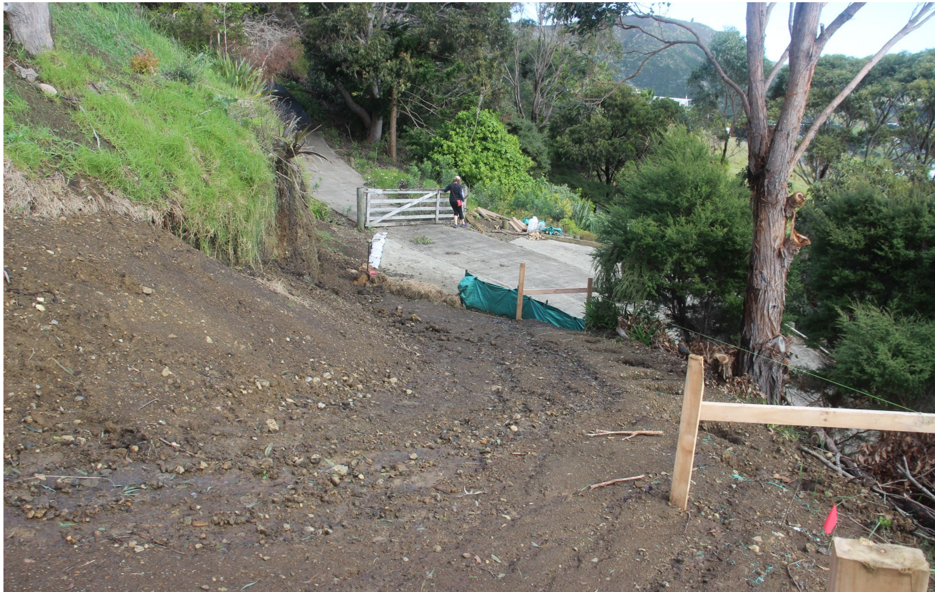
Photo 8: View to south west down proposed driveway to existing concrete driveway
