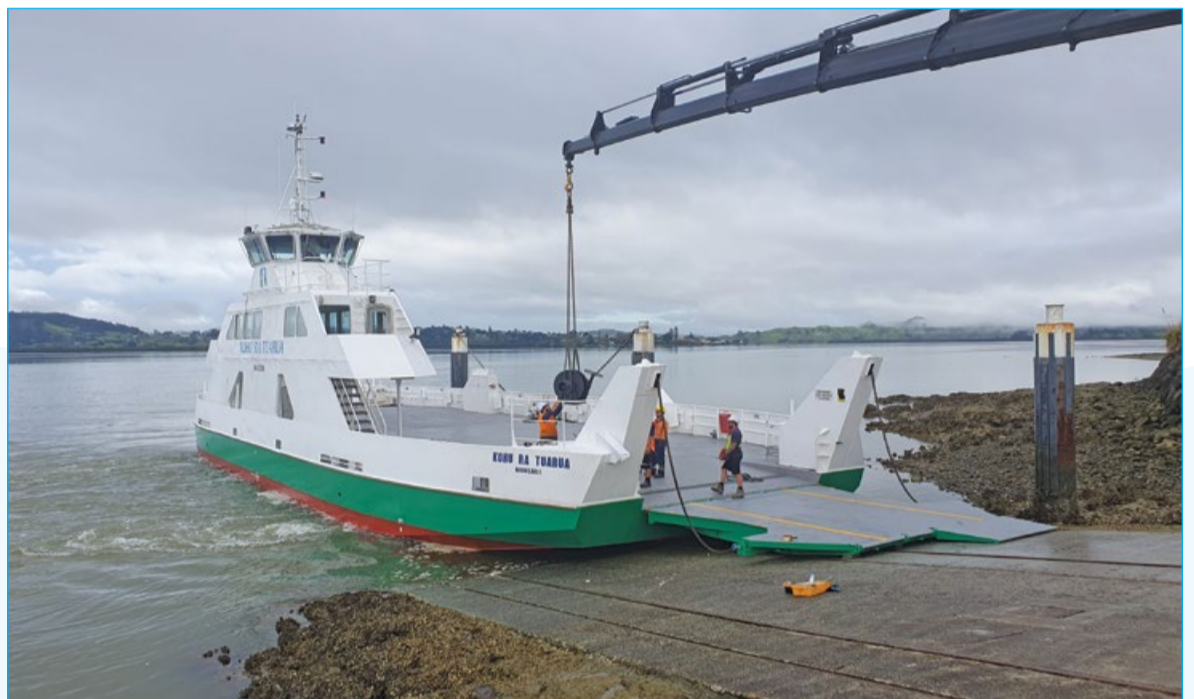
Installing an anchor winch helped complete maintenance work on the 145-tonne Kohu Ra Tuarua vehicle ferry before it resumed operations.
