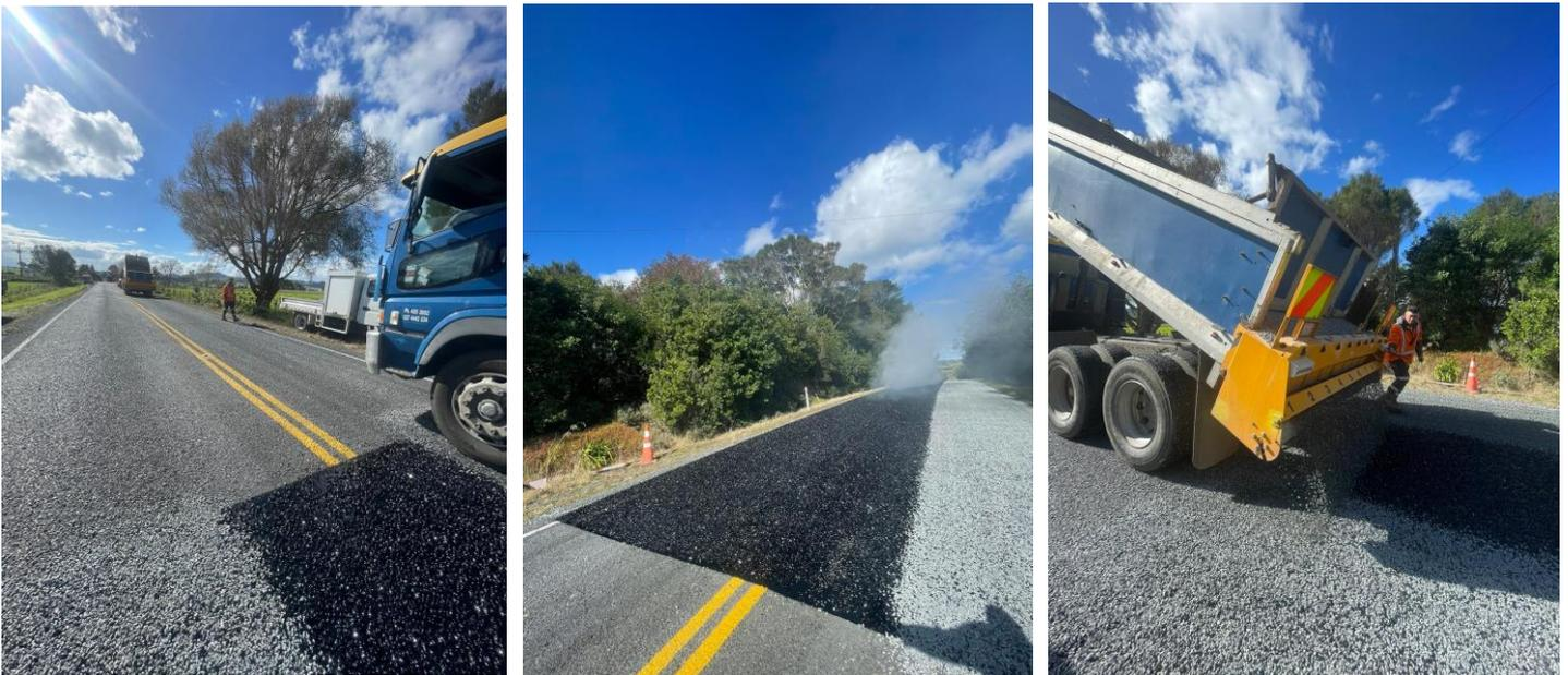
In late April we completed the Asphalt resurfacing of Cobham Road in Kerikeri. This project involved approximately 10,000m<sup>2</sup> of surfacing works along with some additional drainage and shoulder works down towards Kerikeri Inlet Road. A great new asset for the community. See section 25 below for a job where we used the recycled millings!
