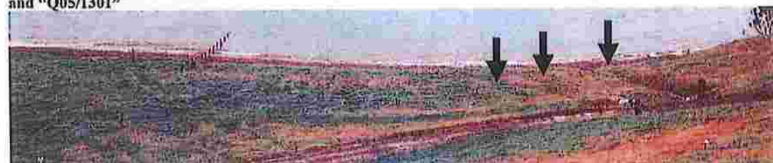
Figure 25. View of proposed house site 9a (now dropped) and Q05/1301 drains
