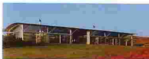
Magnay House – Glenn Murcutt
