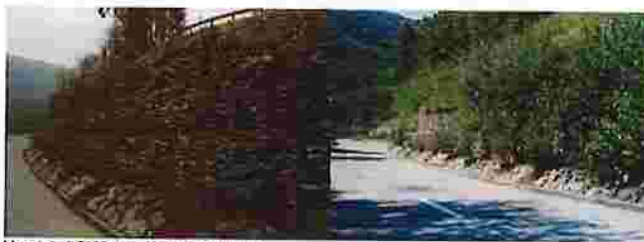
Vegetated Gabions – Winter + Summer
