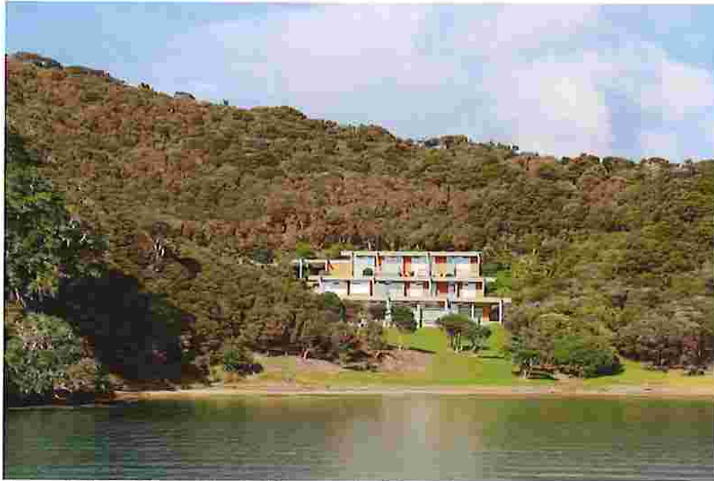
Figure 7: View of the existing built form on Lot 1 from the water.
