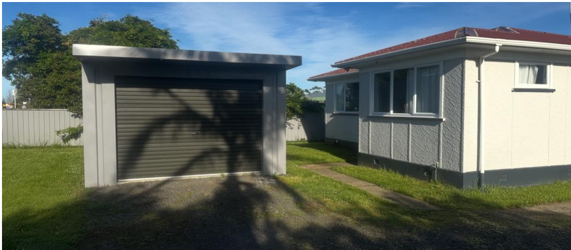
Figure 1 : Southern Dwelling and Garage
