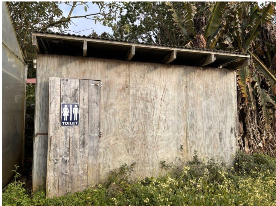
Shed at east end of polyhouse
