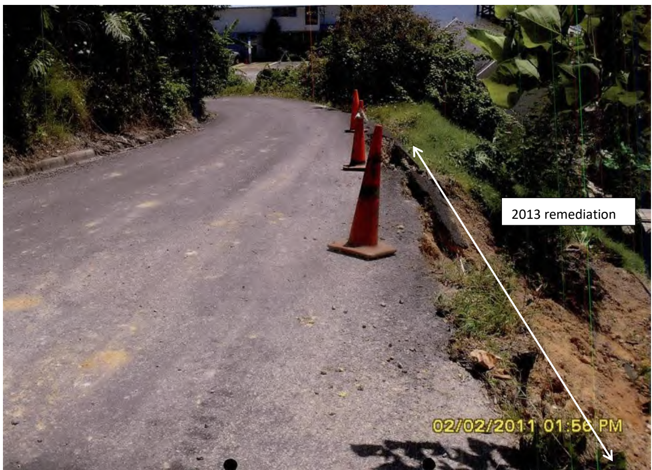
Figure 5 – Undermining/slip on old church road immediately upslope of Whangaroa Community Hall
