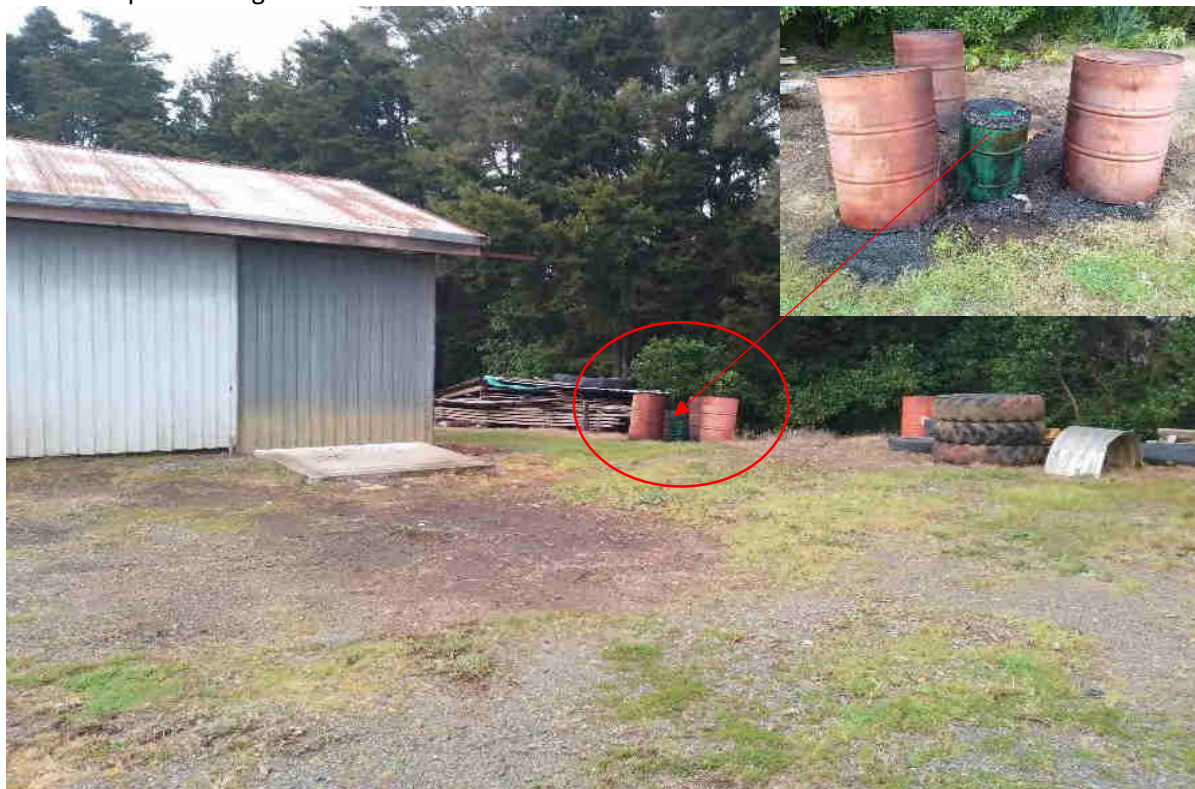
Photograph 3: Central shed (equipment/ storage area). Un-bunded chemical storage. Inset showing localised spill. Looking south.
