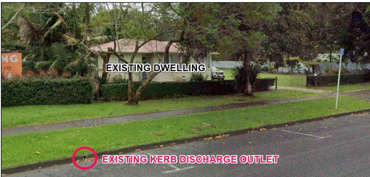
Figure 5: Google Street View – view of subject site from Kerikeri Road, facing north. Existing kerb Discharge outlet shown in bottom left of image.
