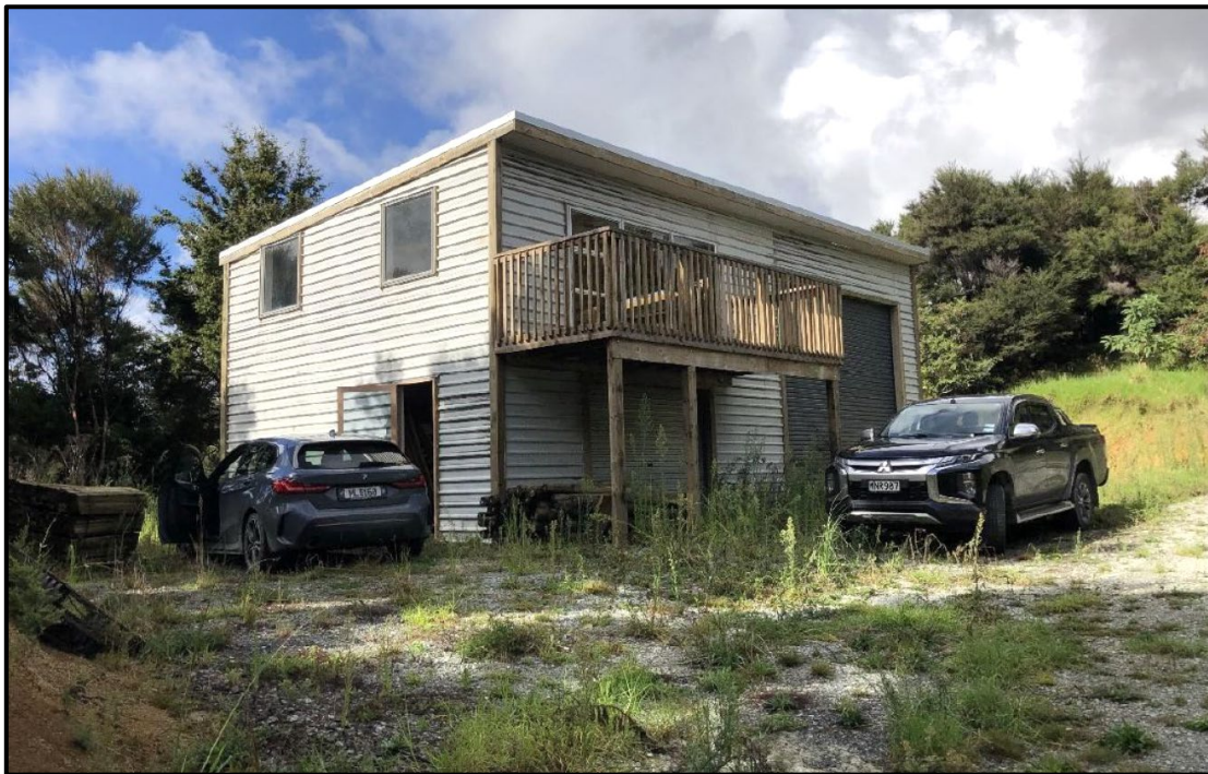
Figure 6: Existing building (northern deck to be removed)
