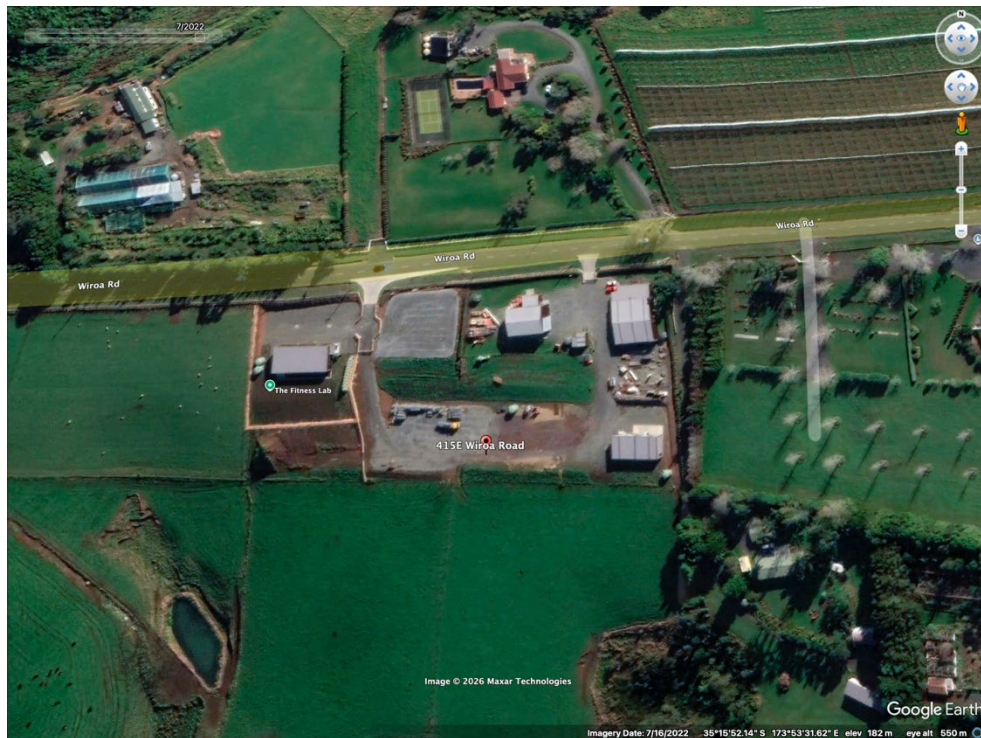
Figure 3 - Site at July 2022
