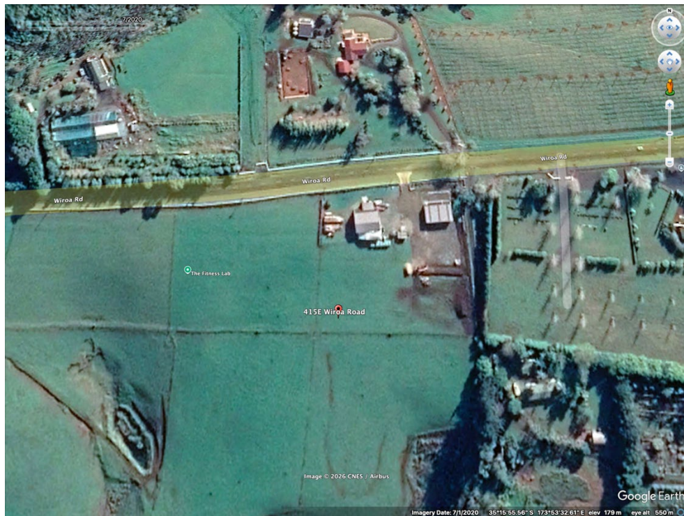
Figure 1 - Site at July 2020
