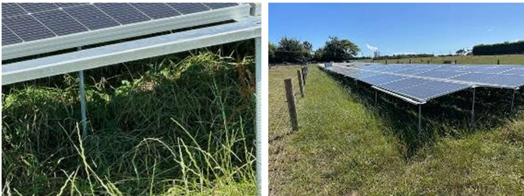
Figure 10: Example Solar Installation and growth eight weeks post-construction.
