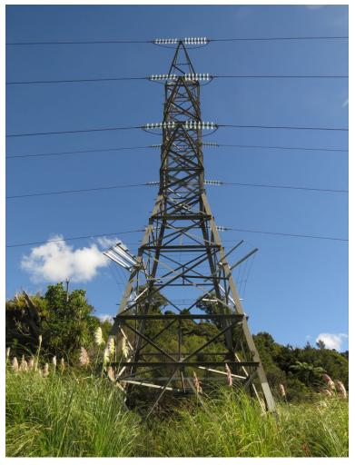
**Figure 1** example of a typical Tower located at Mangamuka West, Site Number B0491 on Top Energy's network. These are usually 22m+ in height.
