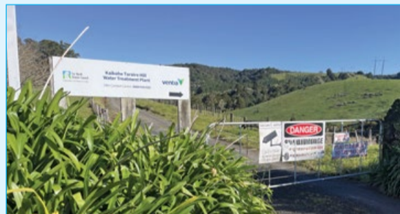
The upgrade will not disrupt the current plant or water supply.
