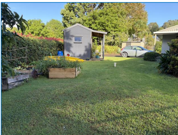
Photograph 2: Location of septic tank and vent on Lot 1.
