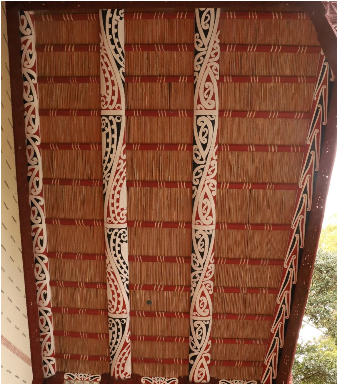
Kōwhaiwhai (proper left) in-situ [2025]
