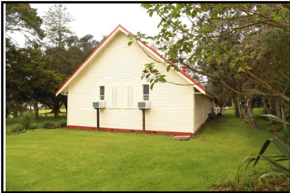
Figure 4 – Te Whare Runanga (rear of building)
