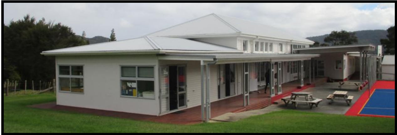
Figure 8 – Existing classrooms along same boundary as proposed new buildings.
